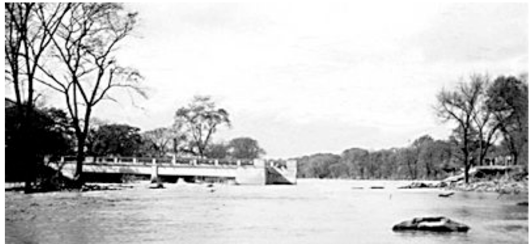
The Lawrence Avenue bridge was washed out by the Humber River
